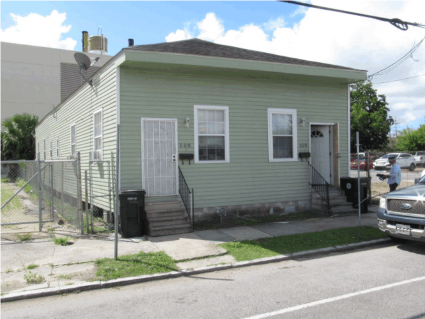
1. Front view of subject property as seen from S. Galvez Street.
